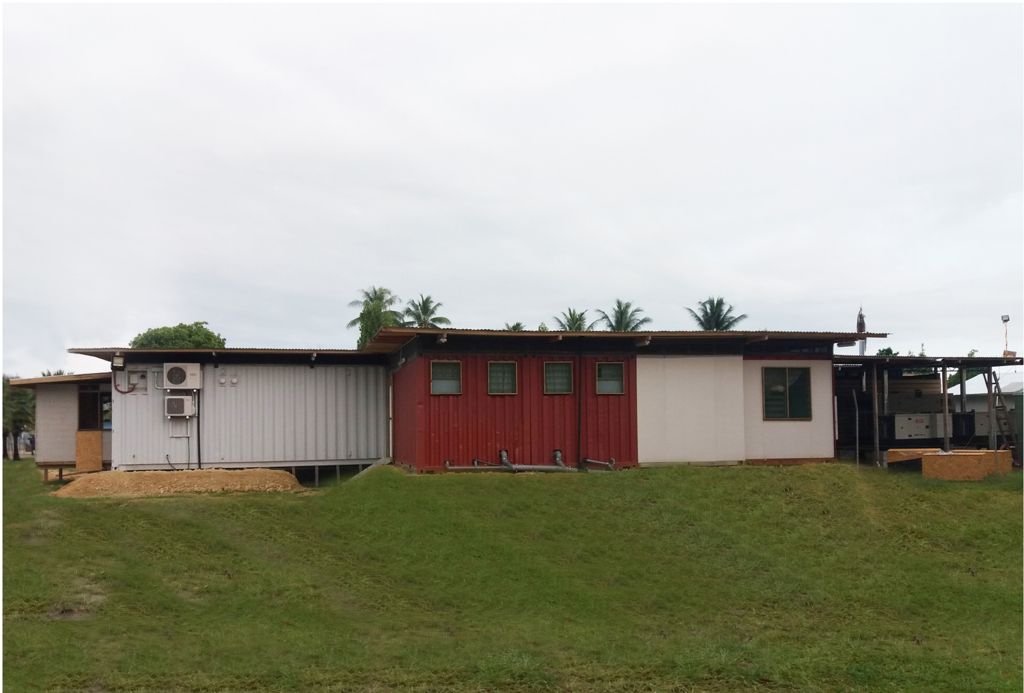
New Modern Boram General Hospital | VAMED Health Project CZ s.r.o. | Papua New Guinea | 2019
