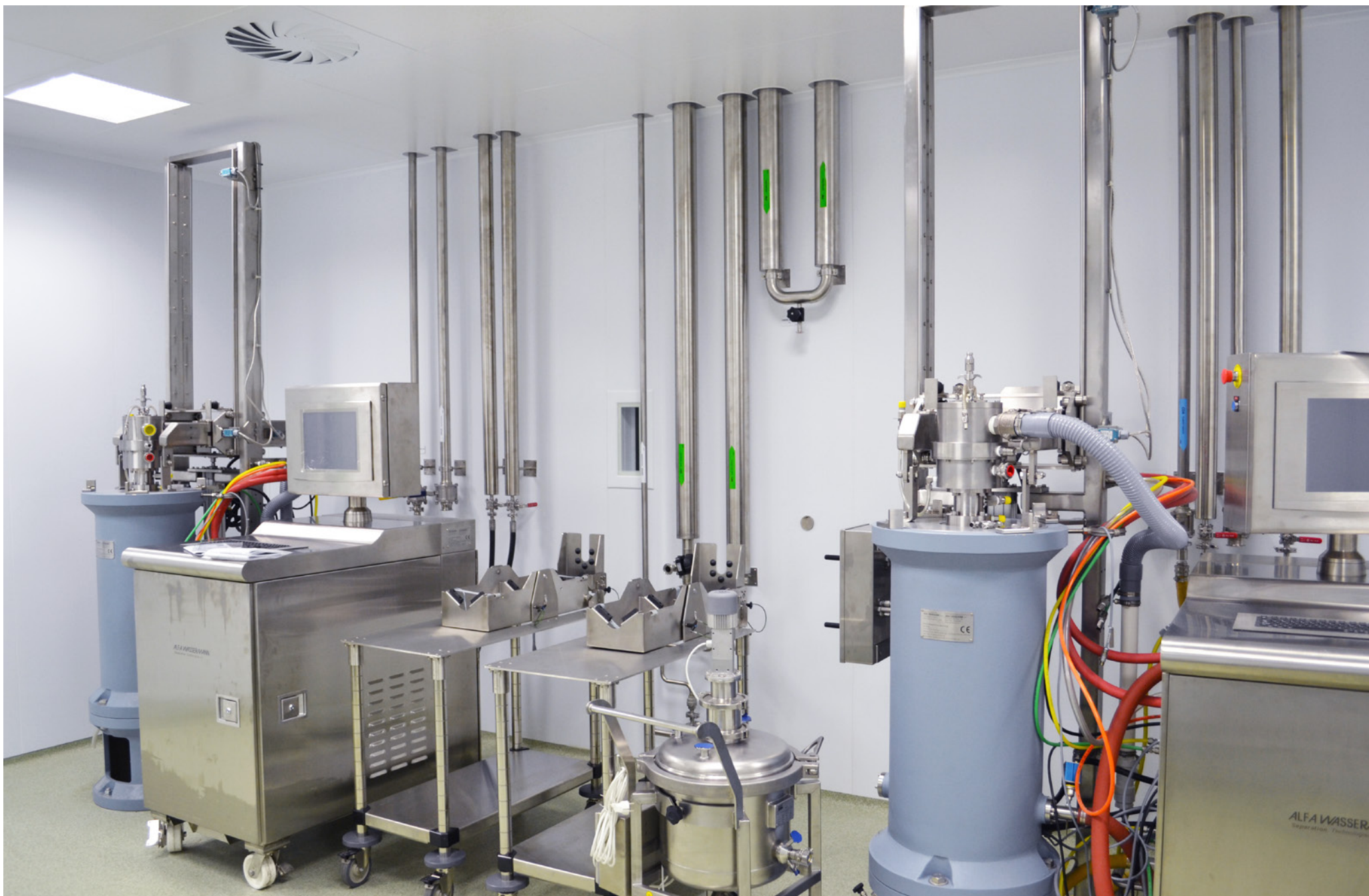
Building B - Development laboratories
