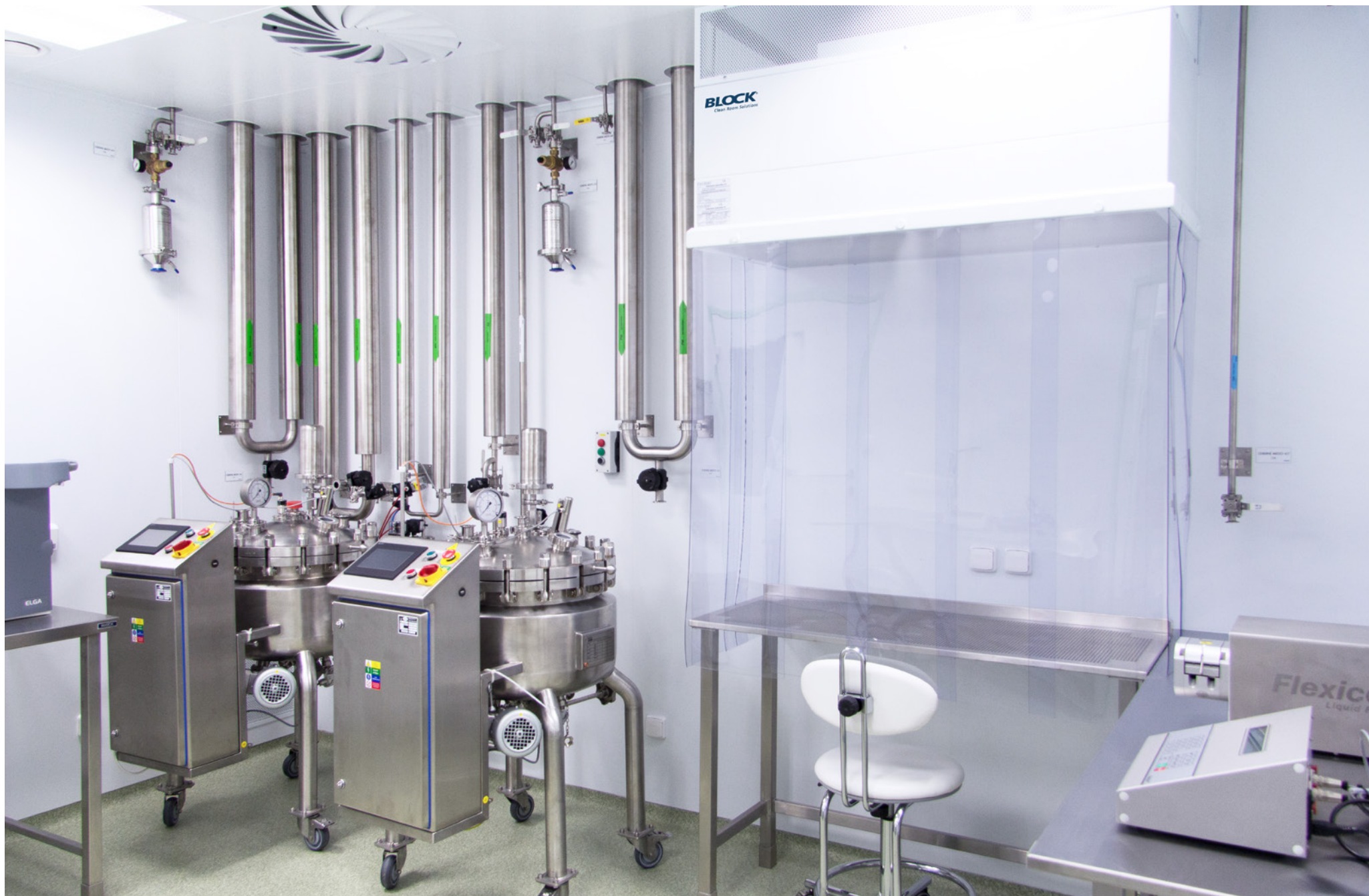
Building A - Research laboratories
