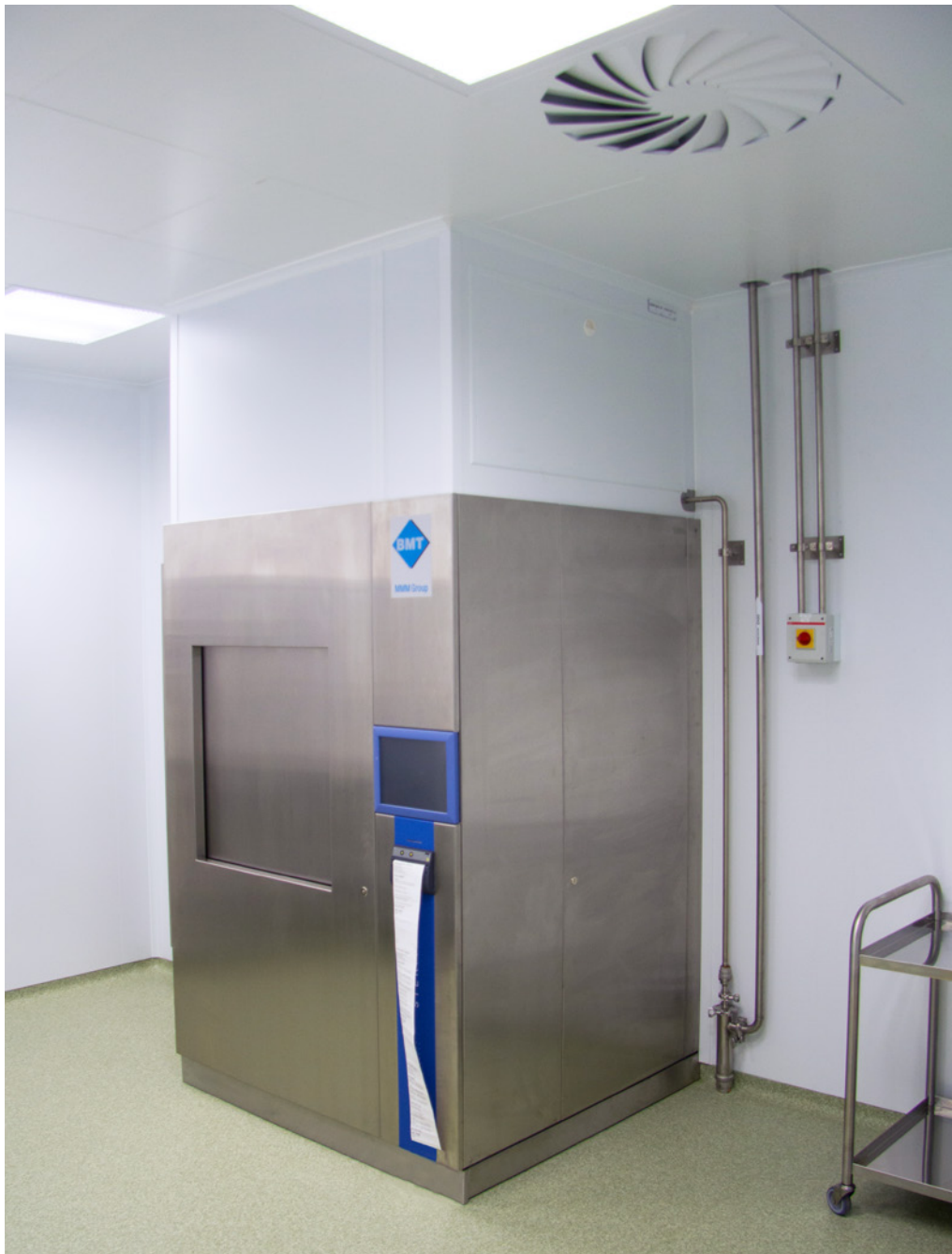
Building A - Research laboratories
